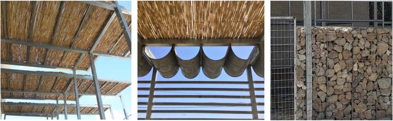
Figure 6, 7, 8. Use of local materials, such as tubulars and bamboo mats, recycled barrels and gabion walls, courtesy of ARCò
