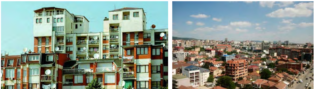
Figure 2. Illegal construction in Pristina (Source: author's photo)
