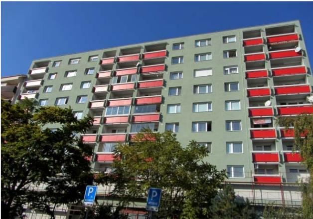
Figure 3: Residential building after realization of thermal insulation – south façade
