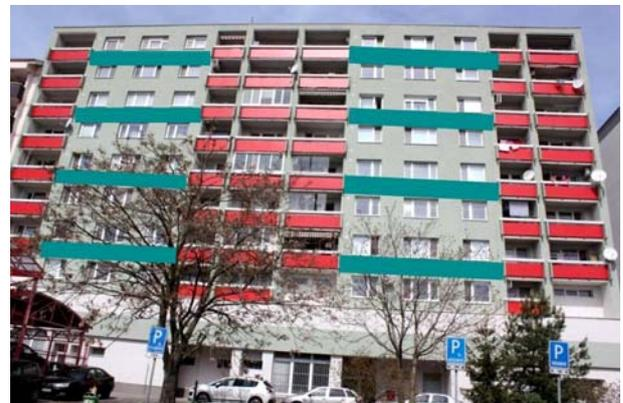
Figure 9. Building with marked application of photovoltaic modules in the place of sill
